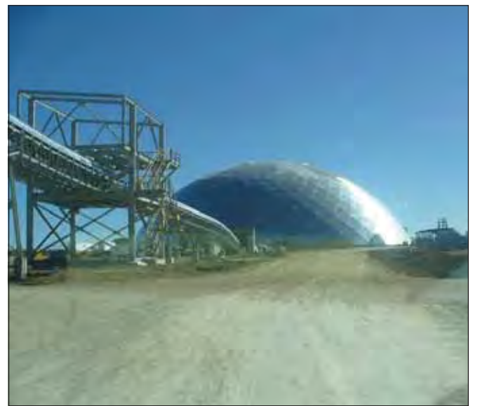
Temcor 78m diameter aluminium dome for limestone storage at the new GCC cement plant in Pueblo, Colorado
