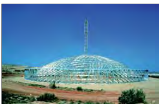
Typical dome construction using Temcor's erection tower method
