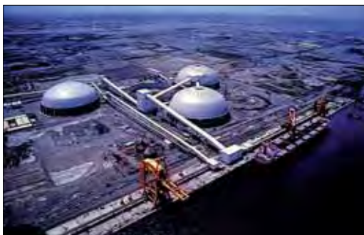
3 of 10 120m coal storage domes, Formosa Plastics, Mai Liao, Taiwan
