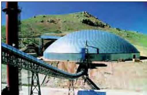
102 meter diameter aluminum dome, Caleveras Cement, Monolith, California
