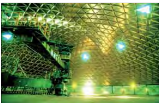
Interior of limestone storage dome
